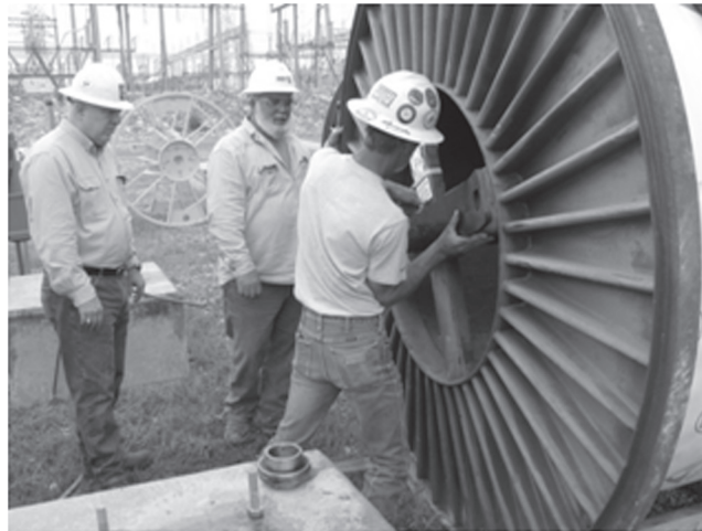
Figure 13. Install Arbor Bar
