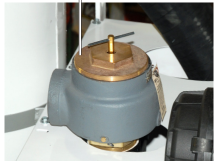
(V11) Collection Tank Pressure Relief Valve (option)
