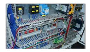
✓ If connectors, cables or other electrical parts show breaks, tears, cuts, are scoured out or show brittle spots, etc., they must immediately be replaced. During these operations, keep the covers of the electrical devices shut.
